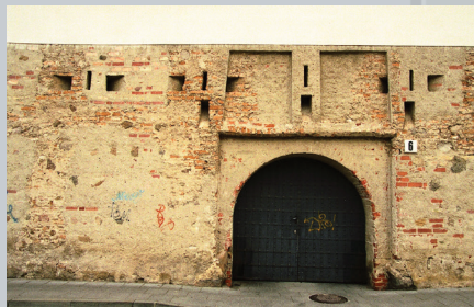
Fragment of the defensive wall built by a citizen in his holding at Šv. Ignoto Street. The firing-slits and the gate have been well preserved. The building standing at this wall was built in the 17 th century. Photo by A. Pliadis.
