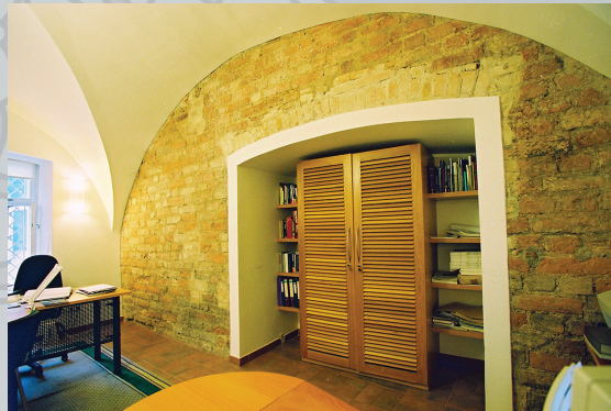
Fragment of the city's defensive wall in one of the offices. Uncovered in 1993. The niche was cut out at the end of the 19 th century. Photo by A. Pliadis.
