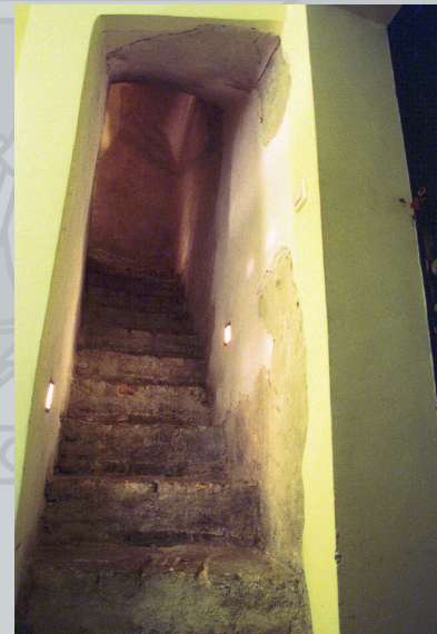
The stairs were made into the first floor. Uncovered in 1999. The vault, steps and plaster on the walls are authentic, dating back to the end of the 17 th and beginning of the 18 th century. The purpose of the stairs remains unknown. They were cut out in the wall at the monastery's main staircase which has not been preserved. In the second half of the 19 th century, most of the staircase was filled with scrap bricks. Photo by A. Pliadis.
